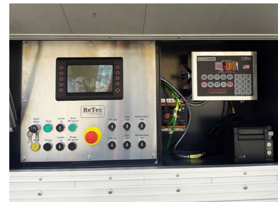
Touch weight- and control panel for plant.
