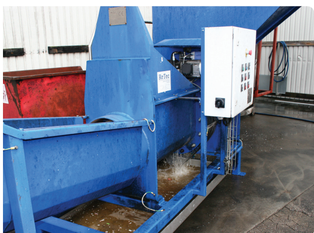
The process is running - the fluid is pouring out
